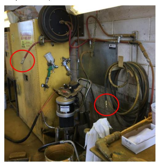
Look at the example above. Which hose is the compressed breathing air hose and which one is general shop air which is not intended to be breathed by a worker and has not been tested for compliance with the CSA standard. A simple label would prevent a misunderstanding and someone using the wrong hose.
